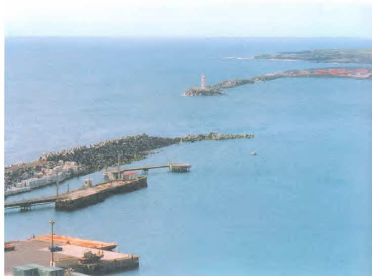
The enclosing breakwaters at Praia da Vitória in May 2003, more than a year after both were breached in easterly storms. The northern arm remains unlit.
