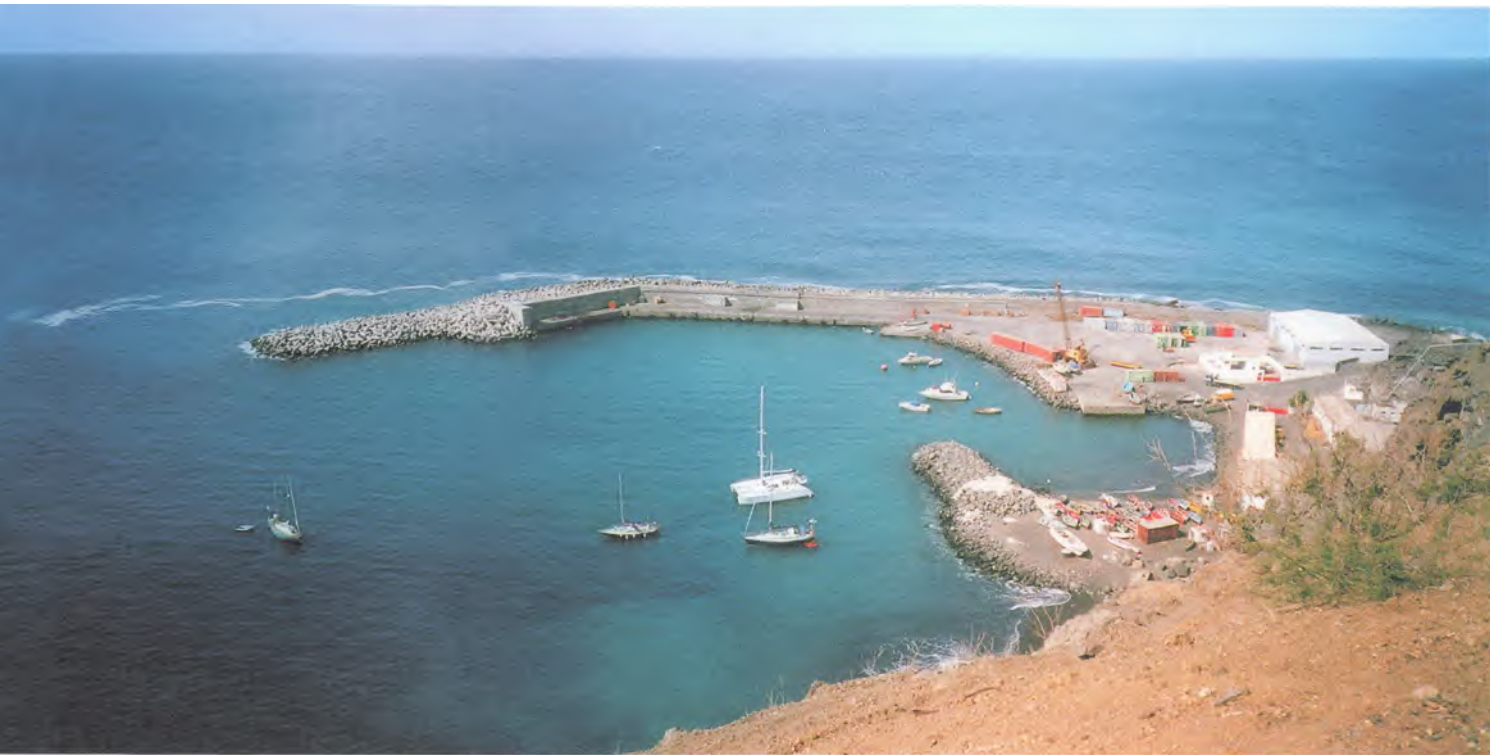
Vale de Cavaleiros, looking slightly south of west. The breakwater was rebuilt and extended in early 2000 after repeated storm damage
